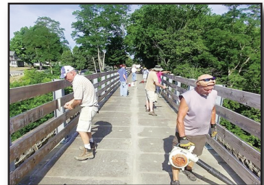
Soon after the S-Curve of the connector was installed, volunteers cleaned the bridge deck and sealed the railings. Seeding of the adjacent landscape will follow.
