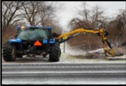
Ditch mowing at Collins...
