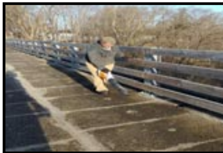
Blowing off the bridge decks, and...
